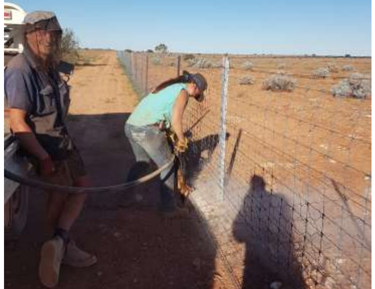
Jillaroo Taylor (New Taylor) Mondy using the air leg to drill holes on the northern netting so we could pin the lapping down, assisted by Eggy The Bullcamel. A day of air legging on the Nullarbor is no mean feat!
