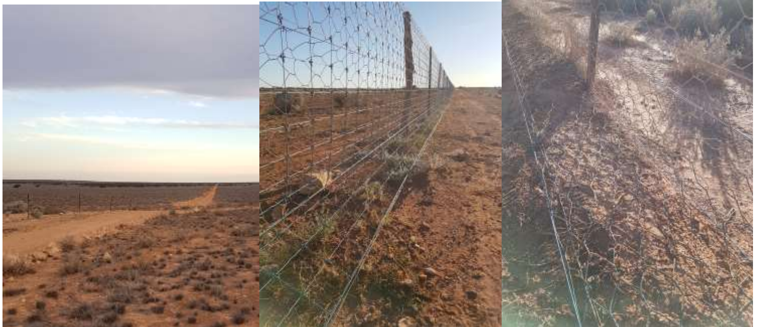
ABOVE: The entire 110km length of the Rawlinna western netting has now been graded with a double cut. This will allow better visibility for patrolling as well as reduce roo and large animal pressure.
