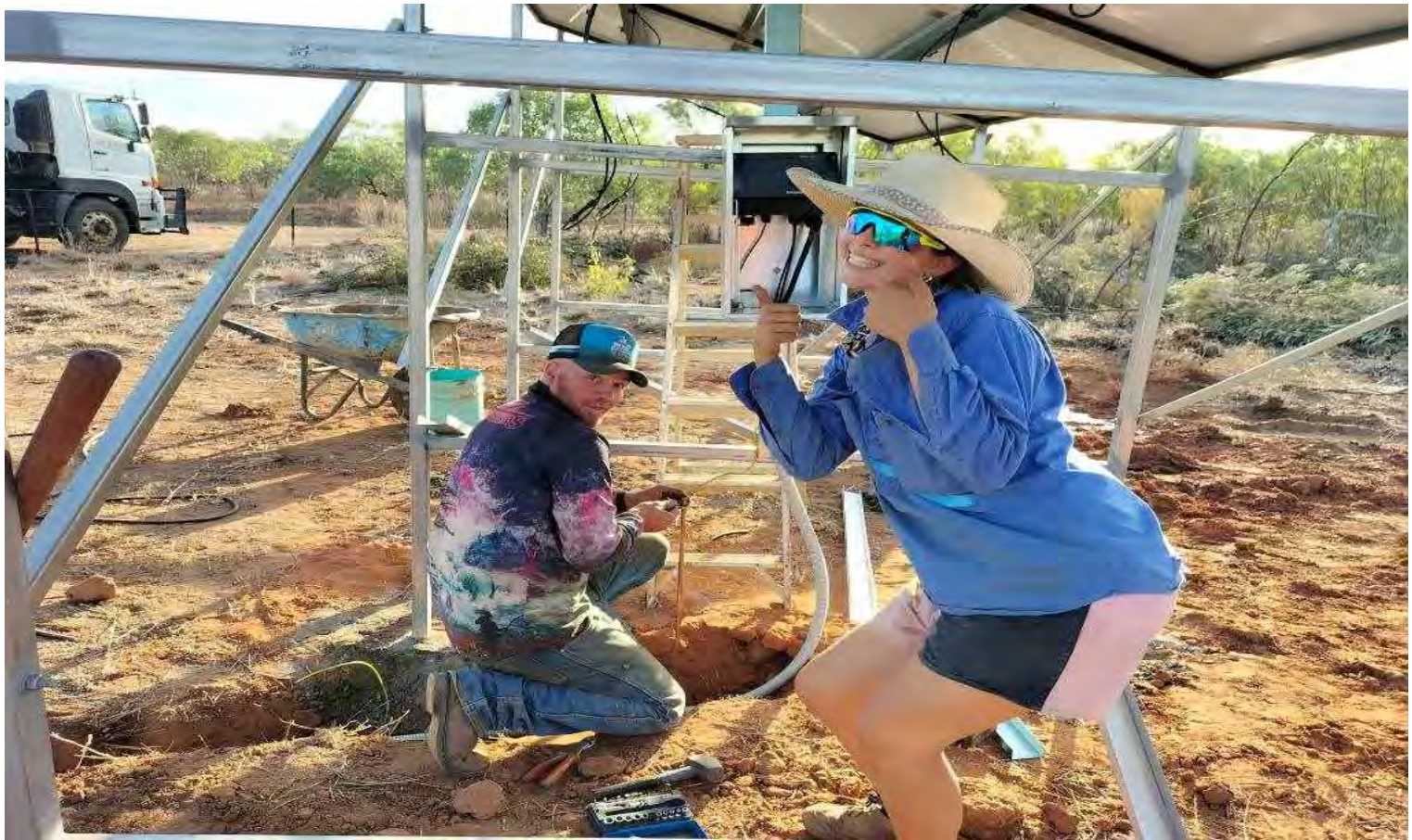
ABOVE: Pup Olsen and Saffie Yates installing solar array at
